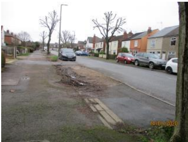
Current highway treatment in front of site and street scene facing north east.
